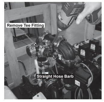
3. Remove the plug from the tee fitting.
