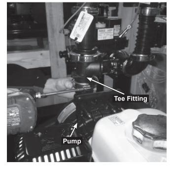
9. Install the cross fitting above the pump in place of the old tee fitting. This may require loosening additional clamps.
